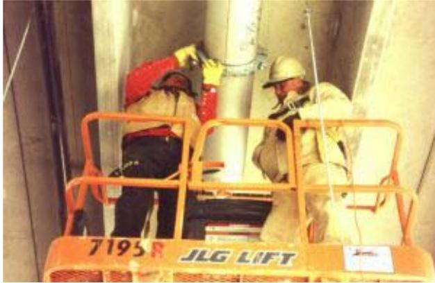
Figure 3. 300 mm drinking water main pipe, light enough to be installed by two people in a new sports stadium in Detroit, USA.
