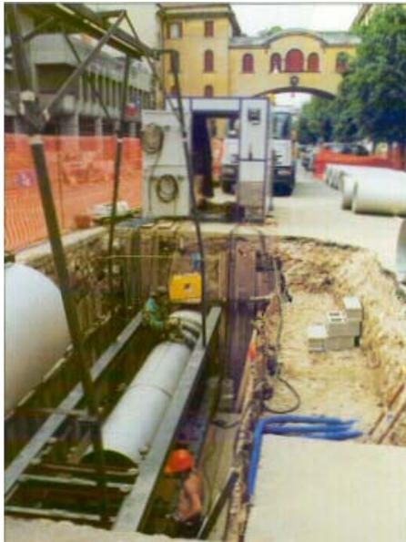
Figure 5. Refurbishment of water main in Padua, Italy using trenchless technology to avoid disruption. Lengths of pipe are orbital welded in the excavation and then pushed hydraulically along the old main.
