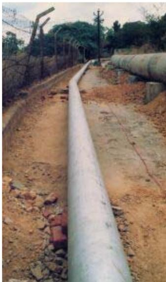
Figure 1. The first use of a stainless steel pipe to handle raw water in India. 300 mm diameter: lower weight meant lower transport and installation costs; no corrosion meant that pumping efficiency would be maintained. Compared with
