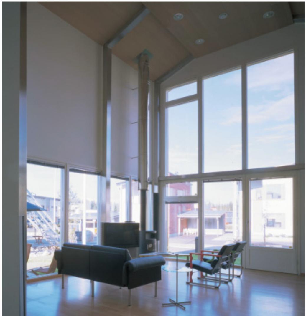
*The shimmering reflection of light on the exposed parts of the stainless steel frame is achieved by polishing the surfaces (grit size 220).*
