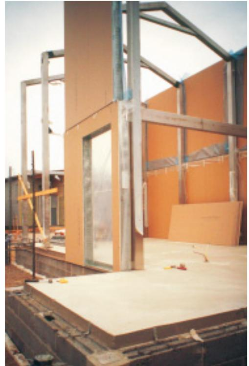
stainless steel hollow sections support the intermediate floor.
