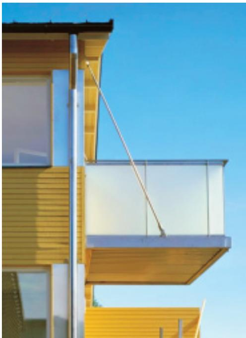
*The stainless steel panels on the façade contrast with the horizontal spruce cladding.*
