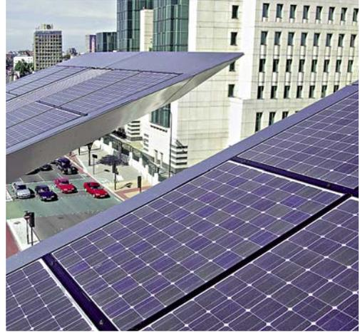
*168 photovoltaic modules are fitted to the top of the cantilevered arms of the roof. Generating around 23,000 kWh of energy per year, they provide around 30% of the bus station's annual electricity requirements.*
