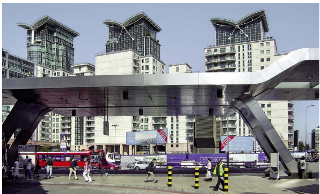
*The broad-spanning frame of the roof is clad with a skin of stainless steel, a material suited to the exacting conditions at this busy inner-city interchange.*
