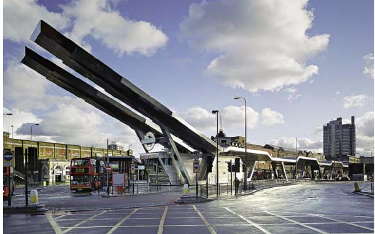
*An undulating strip of stainless steel forms a flowing, continuous roof over the waiting passengers and buses.*
