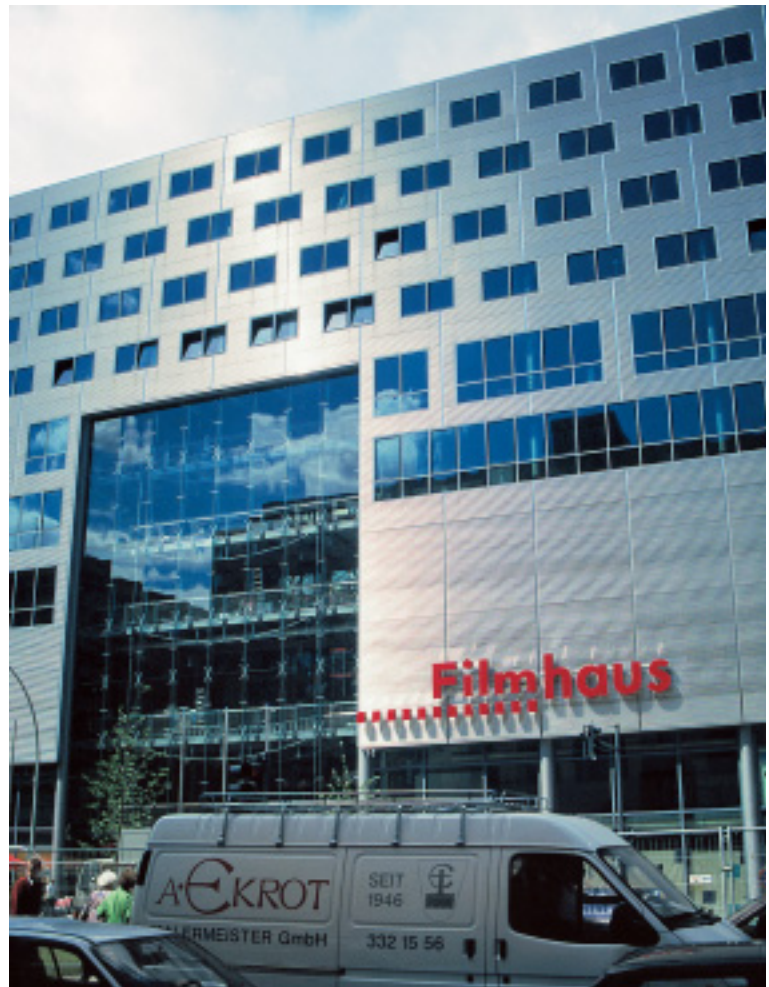
The profiled stainless steel panels articulate and lend structure to the regular, punctuated façade.
