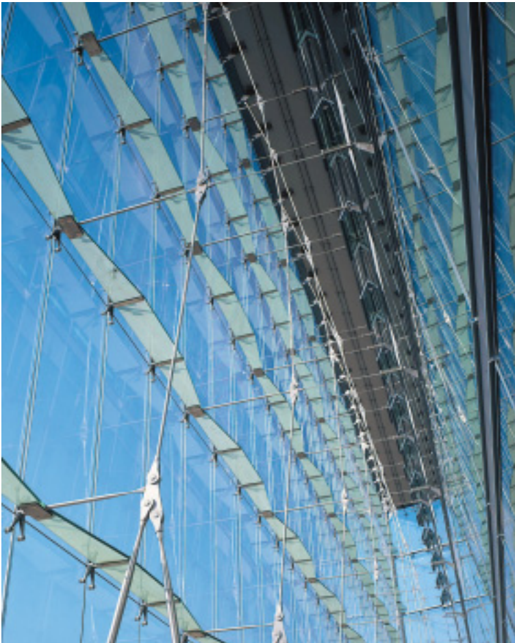
Horizontal glass fins on the inside reinforce the façade structure of stainless steel compression struts and tensile rods.
