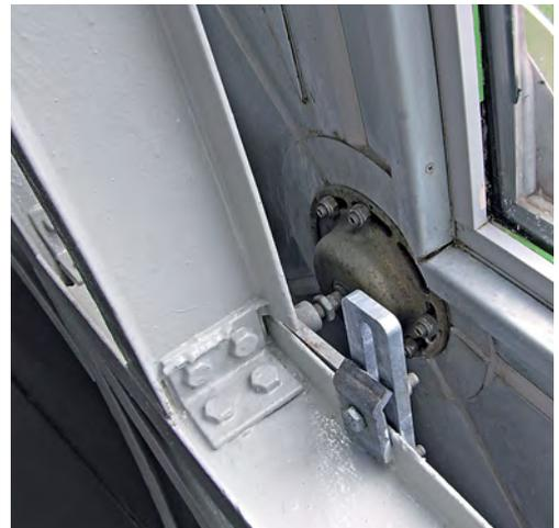
While the new panels were being manufactured, the old aluminium panels were removed and the steel frame of the Atomium sandblasted and painted. In total, there was over 50,000 square metres of steel to treat. Some components had to be strengthened or replaced and it was necessary to fit new connection pieces between the tubes and the spheres.
