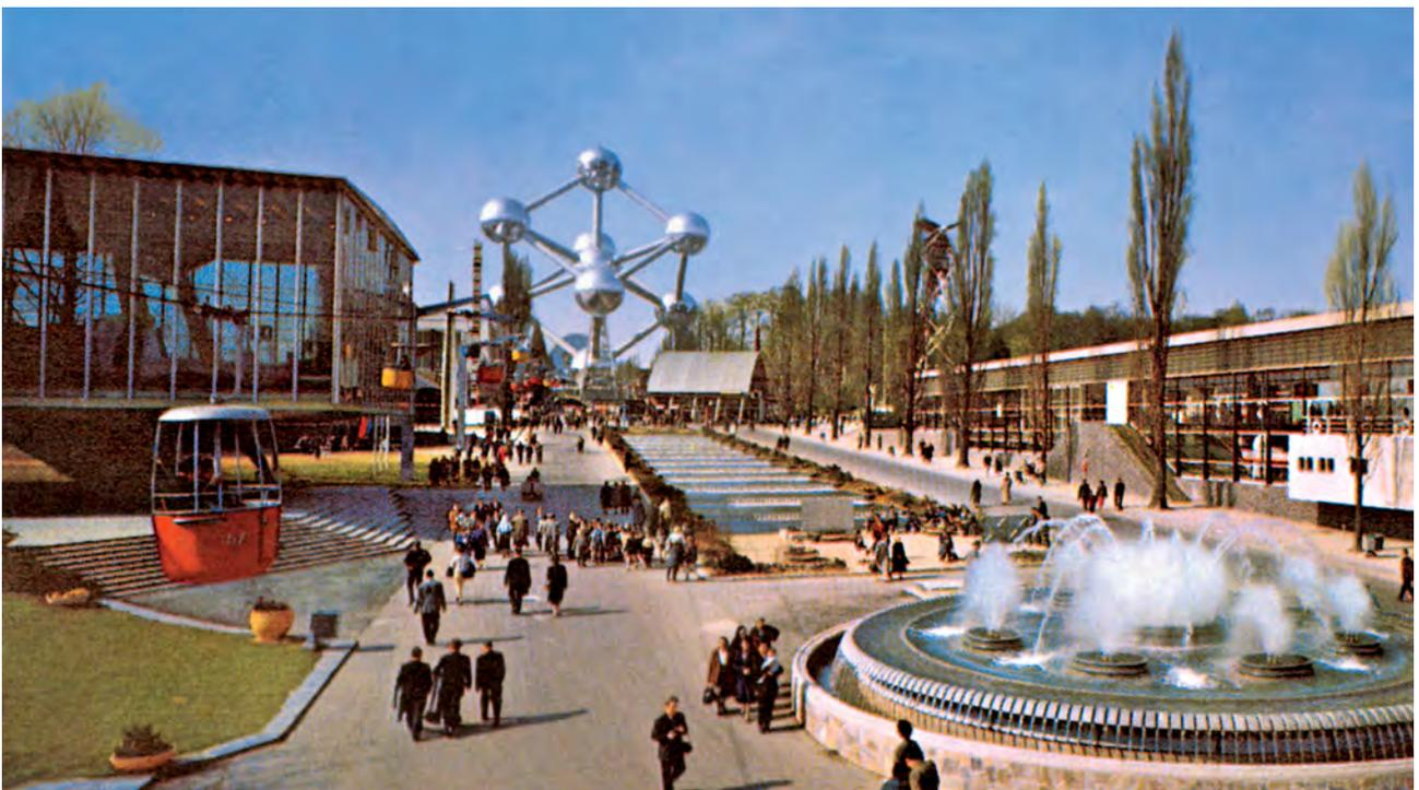
central tube, but for structural reasons, it was necessary to support three of the spheres on lattice-truss columns (I1, I2, I3).
