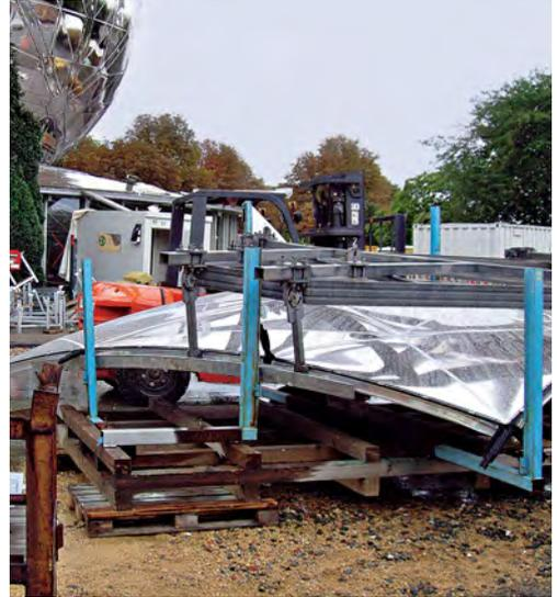
*The curved triangular sandwich panels were manufactured in the workshop and transported to the construction site.*
