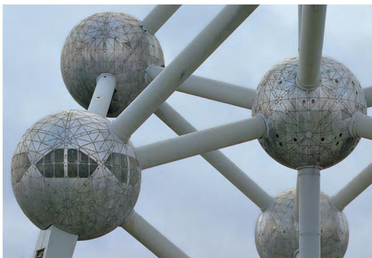
The curved panels that make up the new skin are a 10-cm thick sandwich construction of 1.2 mm stainless-steel sheet, an insulating core of rockwool and 1 mm galvanized steel sheet. Only the three spheres (M1, M2 and M3) that are not used for structural reasons were fitted with non-insulated cladding of stainless steel. Thermal-break aluminium profiles connect the stainless and galvanized steel sheet of the sandwich panels. To prevent galvanic reactions between the three
