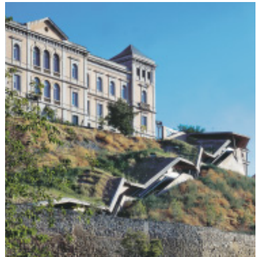
The escalator system is divided into six parts, following the topography of the hill. It bridges 36 metres in height.
