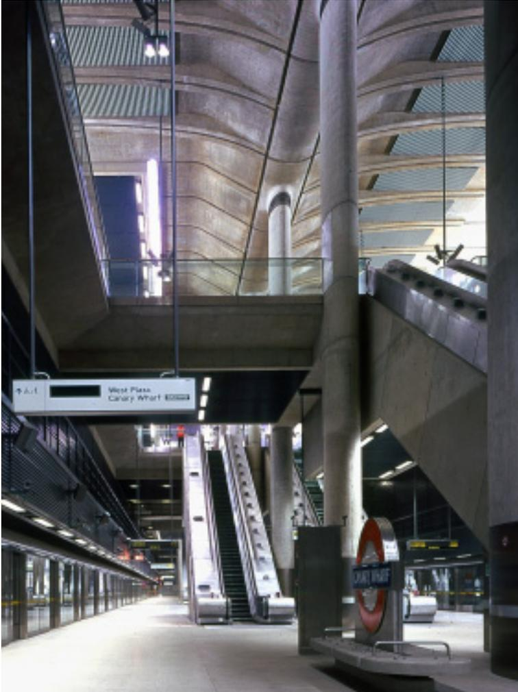
*Lifts have transparent glass sides to enhance passenger security and deter vandalism. Fire resistant requirements (zero gas emission tolerance), as well as scuff resistance were the guiding considerations in specifying stainless steels for the lift panels and escape route gantries, in 2 mm thick type 1.4401 (X5CrNiMo17-12-2).*
