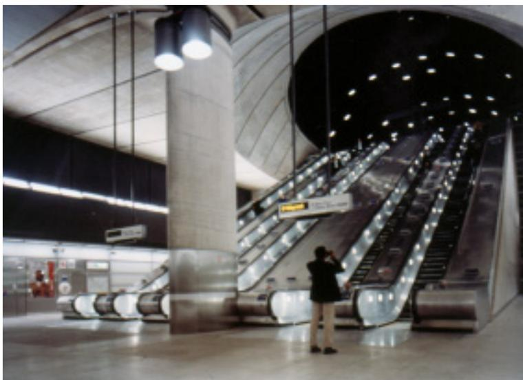
*Foster and Partners used a simple palette of hard-wearing constructional materials – unadorned concrete, glass, and stainless steels. This robust aesthetic is most pronounced at platform level, where satin finish stainless steel clads the oval-section columns in a critical damage-prone area.*
