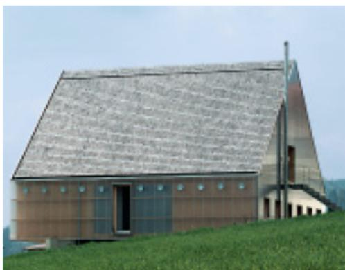
*The exhaust gases from the wood-fired central heating system in this detached house are expelled through an external, double-walled chimney of stainless steel. The material itself and the high quality of workmanship ensure many years of trouble-free operation.*
