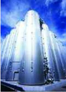
*One solution to the age-old problem of the corrosion of soy fermentation vessels is to make new plant out of a super austenitic stainless steel (in the case of these tanks a proprietary grade with 23% chromium, 25% nickel and 5.5% molybdenum).
