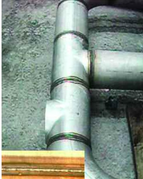
*The heat-tint formed on stainless steel welds must be removed by pickling to restore the material's excellent corrosion resistance.
