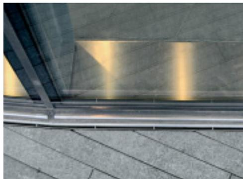
*For the Greater London Assembly a special façade drain with narrow slot was developed, in high-gloss stainless steel. This system, designed to run along curved or straight façades, drains away water from the building both efficiently and unobtrusively.*
