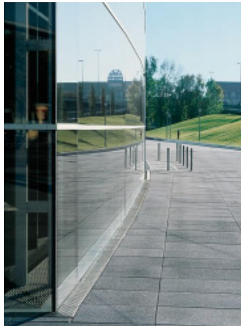
*Provided the right grade of stainless steel is used, drains and drain covers have high resistance to frost and de-icing salts as well as to the chemicals used during façade cleaning.*
