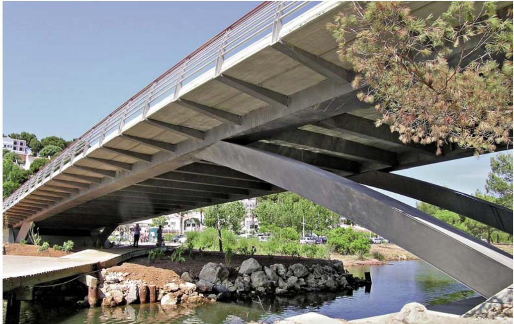
*A pickling paste was applied to the stainless steel frame after welding, to remove discoloration and scale. The unified matt surface structure was achieved by subsequent beadblasting.*
