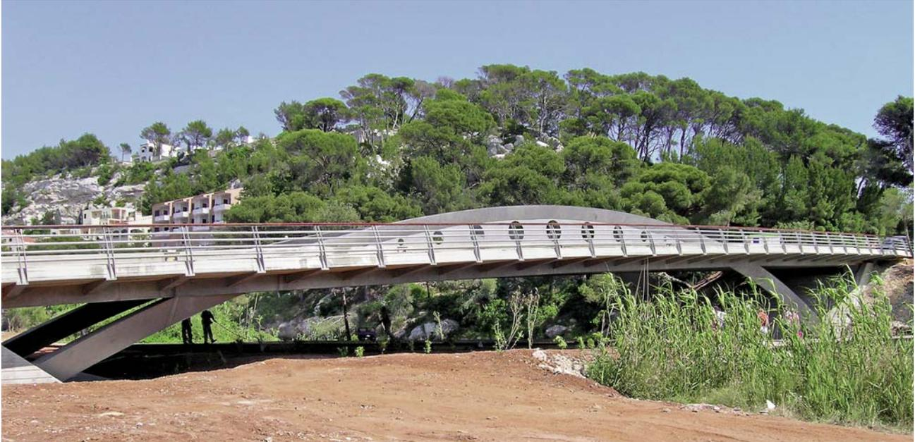
*The inclined struts between the outer ends of the arches and the longitudinal beams take up the horizontal forces in the arches, thereby relieving pressure on the foundations.*
