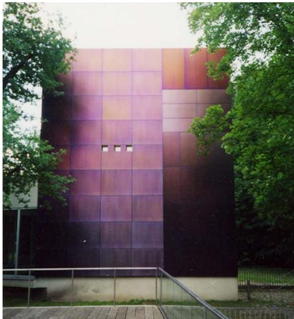
The sheeting panels were simply riveted to the sub-frame using stainless steel rivets and mastic applied to seal the panel joints. Since erected about 25 years ago the panels have only been rain washed. No visual staining of the panels was apparent when the building was viewed in 2000.
