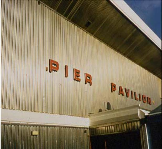
From the shore end of the pier, the pavilion is attractive and displays the familiar stainless steel sheen. At close range (2m) some staining can be seen, particularly on the upper cladding directly under the overhang, and on the walls facing the ocean. Almost certainly, the stains are the result of salt deposited from sea-spray that dry out on the steel. This staining is considered, however, to be superficial and could be removed by cleaning if desired.
