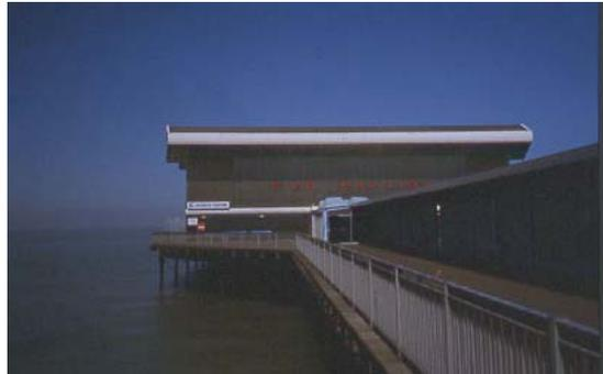
The sports pavilion was built in 1976 at the end of the pier at Herne Bay, a part of the Kent coast that juts out into the North Sea. Clad with trapezoidally profiled stainless steel sheeting, the building was designed to be free from routine maintenance, and, after 26 years of exposure to the marine environment, no maintenance has so far been carried out.
