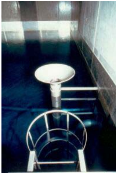
Figure 4. Reservoir in Italy lined with stainless steel. Courtesy of Centro Inox.
